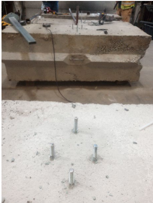
Bolt Setting for Market Shade Blocks
