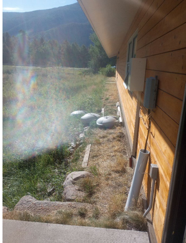
Debris Cleanup at MFC
