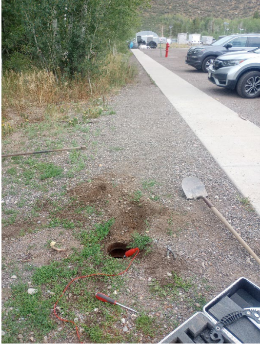
Maloit Park Water Shut Off for WTP Tie-In
