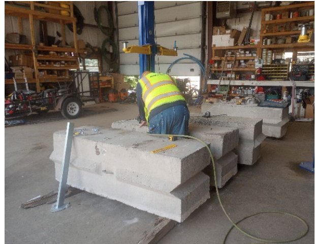
Anchor Bolt Hole Drilling for Market Shade Blocks
