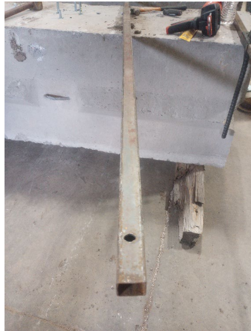
Water Main Line Key Fabrication
