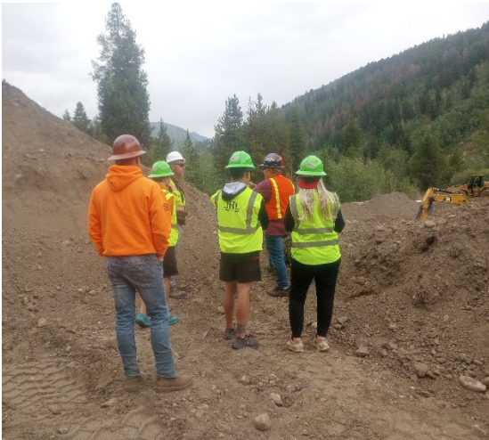
Council WTP Site Visit 7/29
