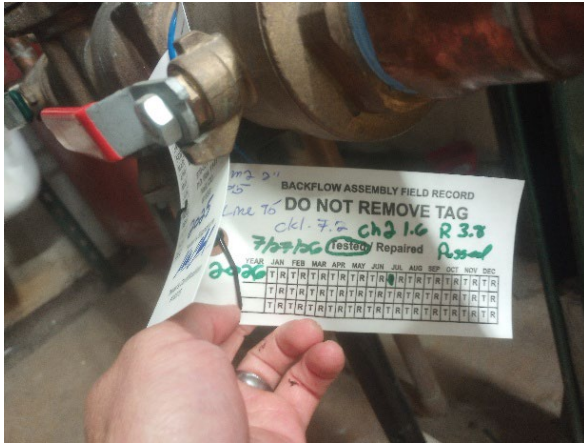
Town Hall Backflow Testing
