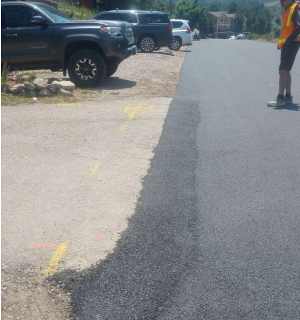
Taylor Ave. Driveway Repairs
