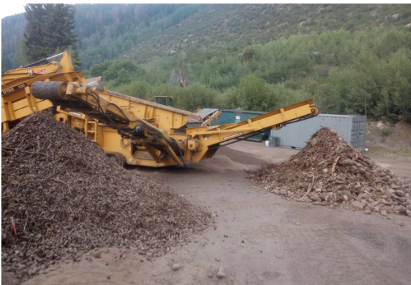
Sediment and Material Screening at WTP
