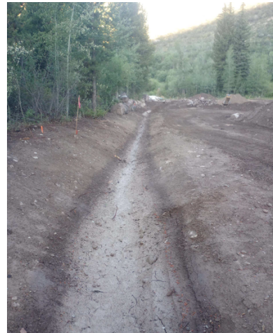
WTP Perimeter Drain
