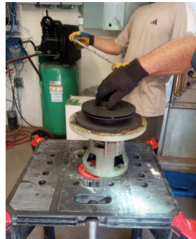
Glycol Pump Repair at PW Shop
