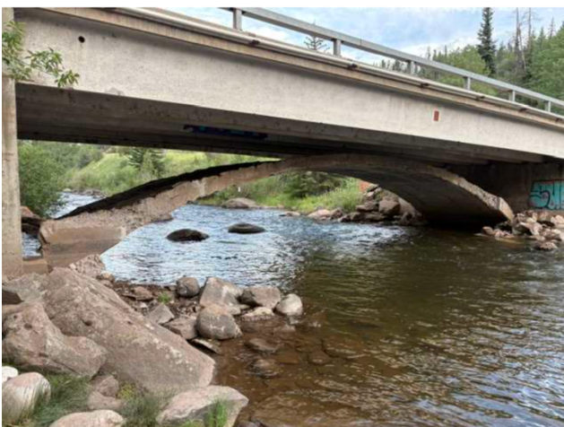
Sides and overlying material removed.
