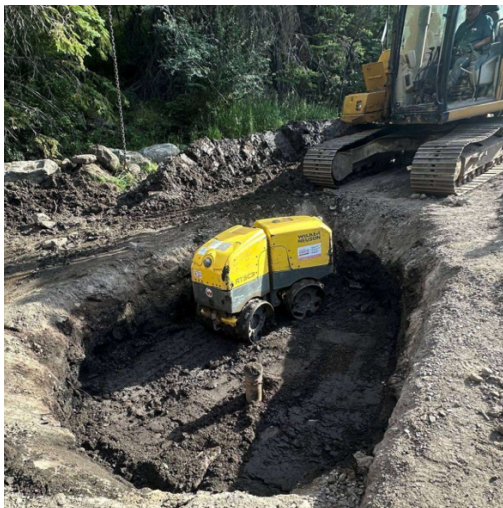
Filling and Compaction
