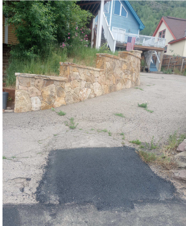
Taylor Ave. Driveway Repair
