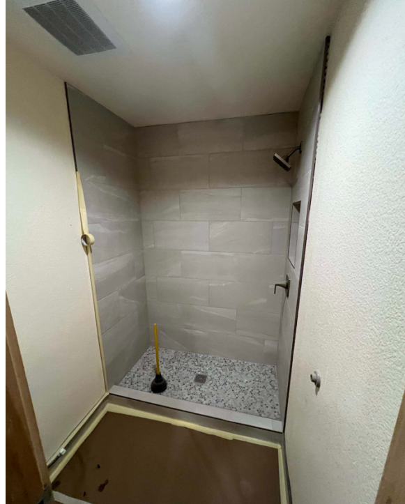
Tile Shower Nearing Completion
