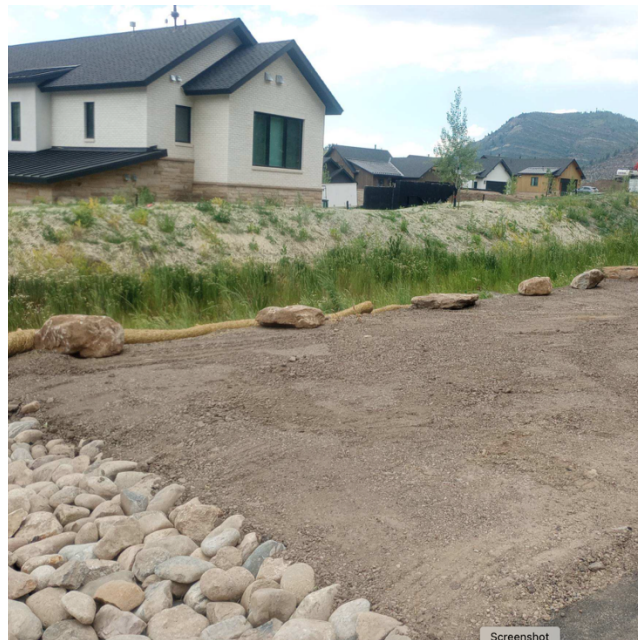
Taylor Ave. Boulder Relocation
