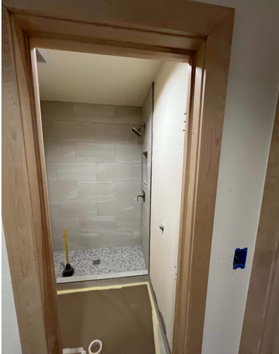
Bathroom with New Shower
