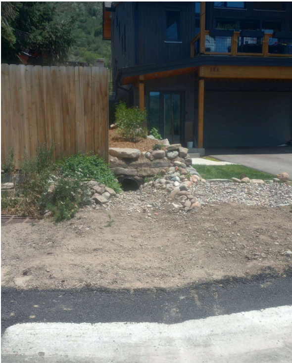
Taylor Ave. Drainage Work
