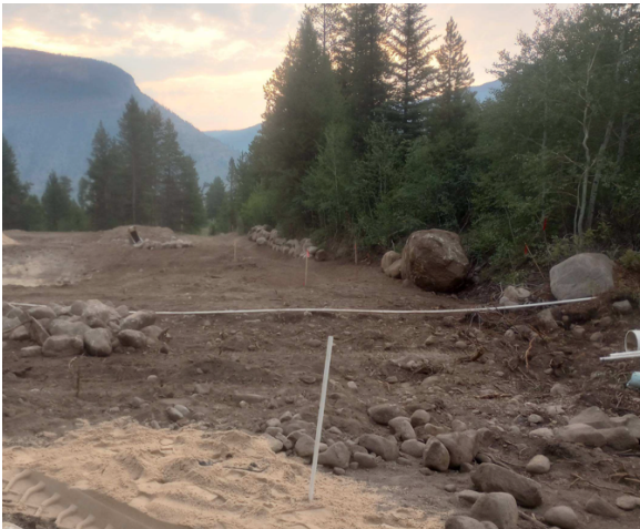
Water Treatment Plant Construction
