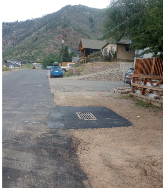
Taylor Ave. Drainage Work
