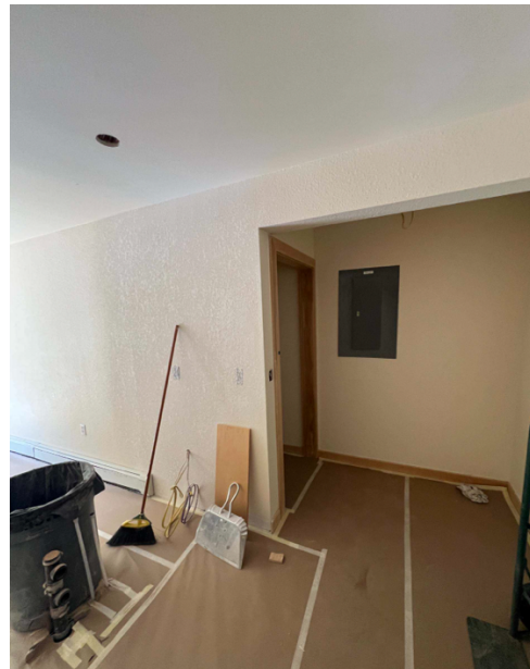
Apartment kitchen area.
