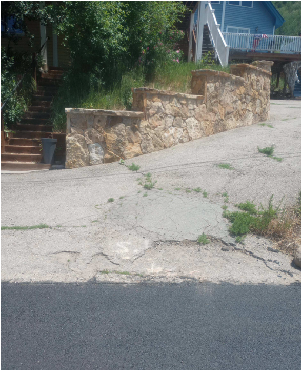
Taylor Ave. Driveway Repair
