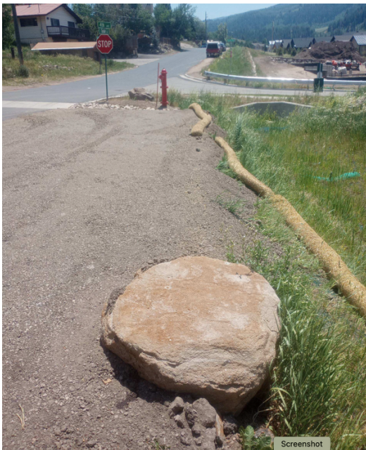
Taylor Ave. Boulder Relocation
