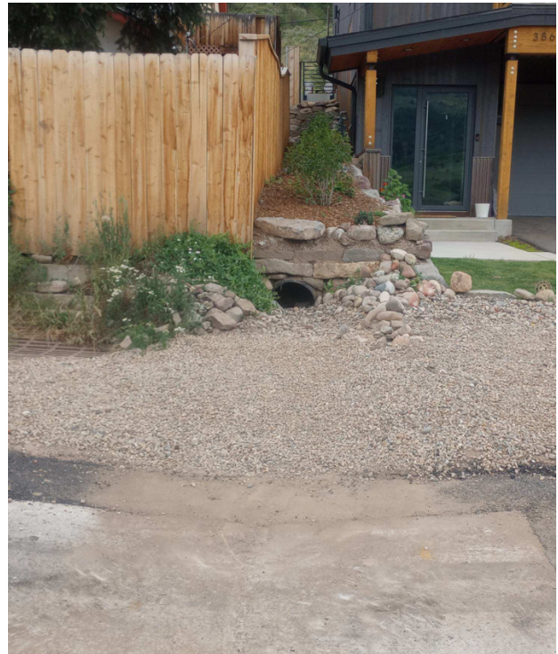
Taylor Ave. Drainage Work
