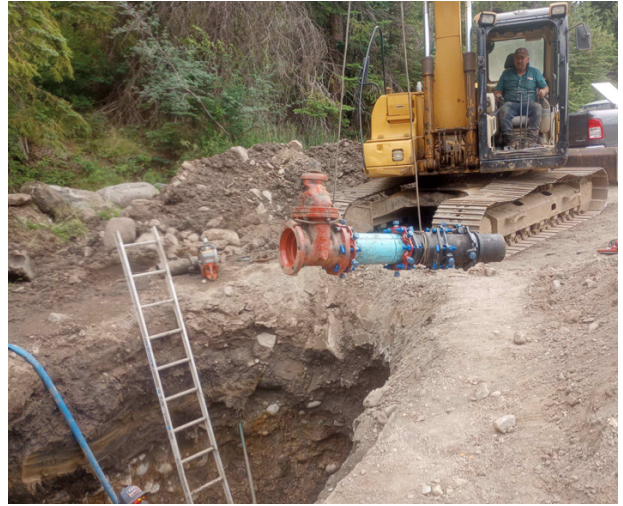
New Valve and Line Replacement
