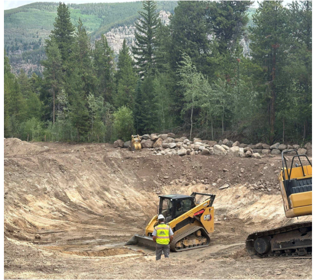
Water Treatment Plant Construction
