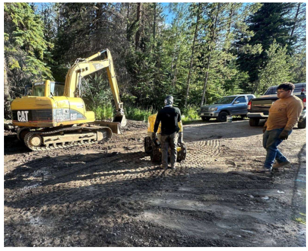
Final Grading and Compaction
