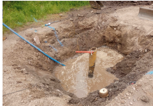
Mail Line Excavation
