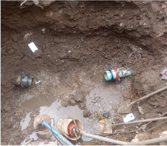
Main Line Valve Removal
