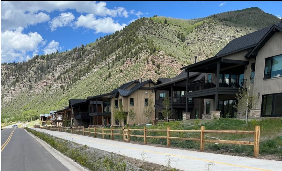
-Photo Credit: Kevin Rindy, Town of Minturn -Figure 2: Photo from Town Staff showing the Fence that was installed.
