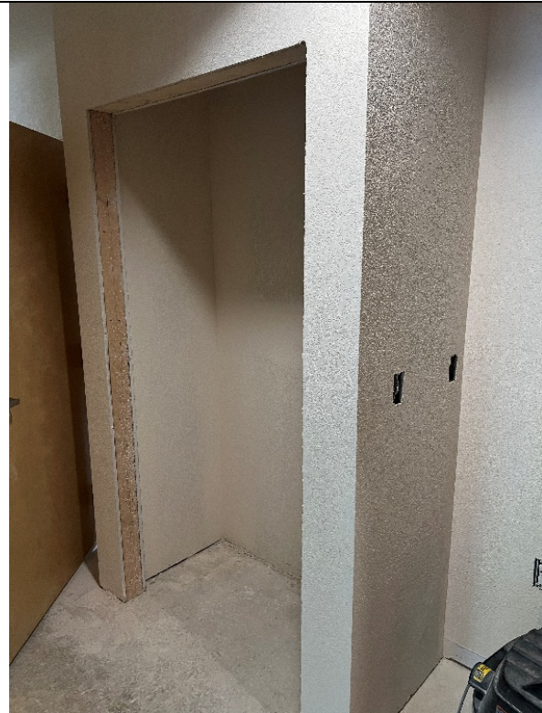
Future storage closet. (Former office door location)
