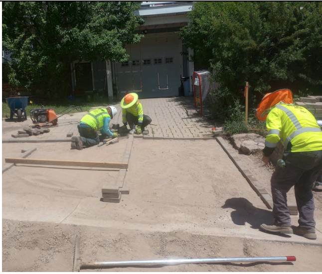
Driveway repair work on Taylor Street.
