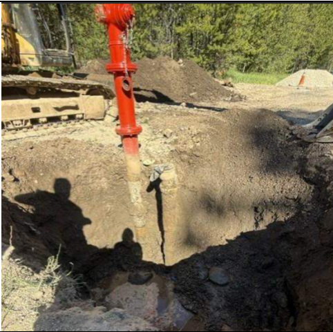
Area of excavation around fire hydrant.
