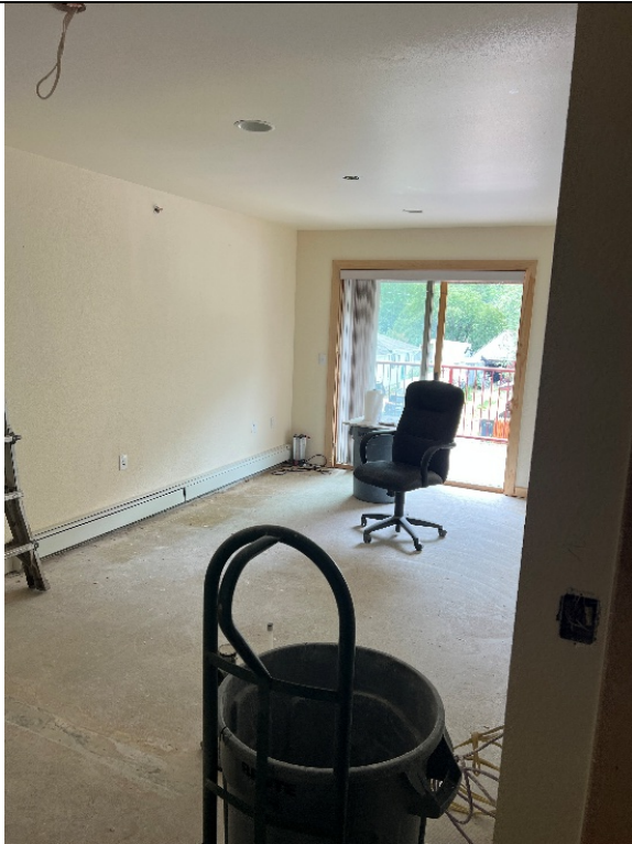
Restored living room area.
