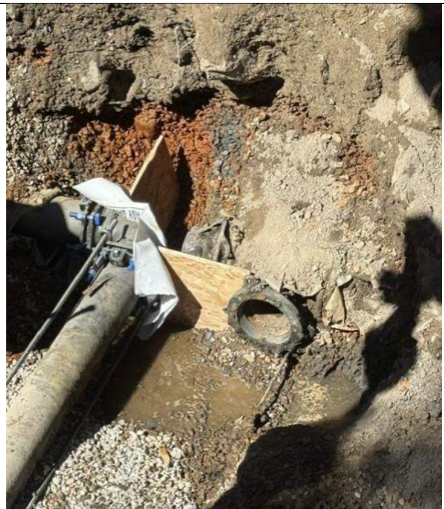
Water main work for 491 Main Street.
