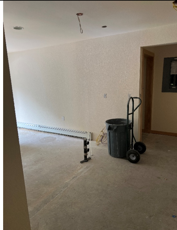
Removed office wall for living room area.
