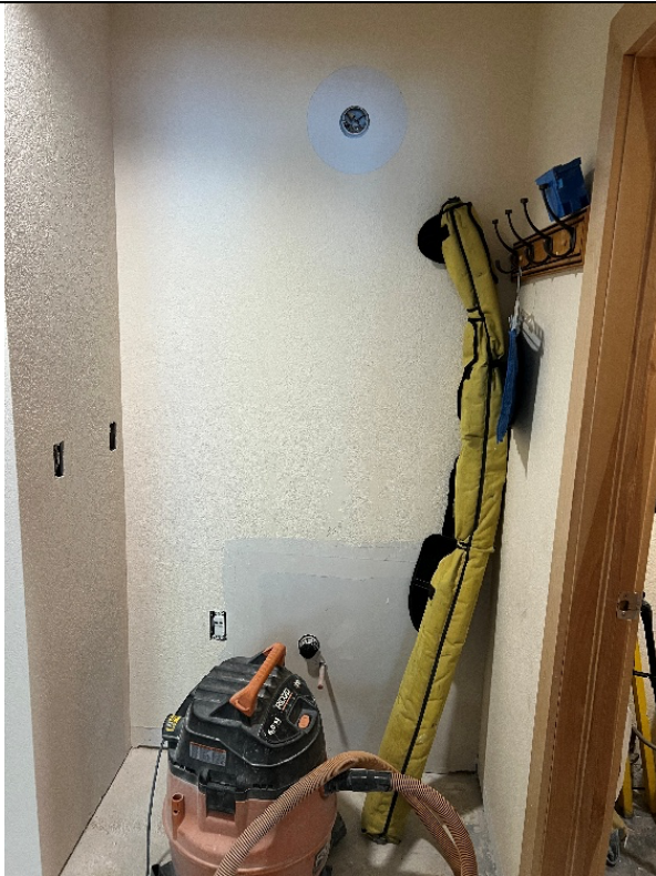
Future bathroom sink and vanity.
