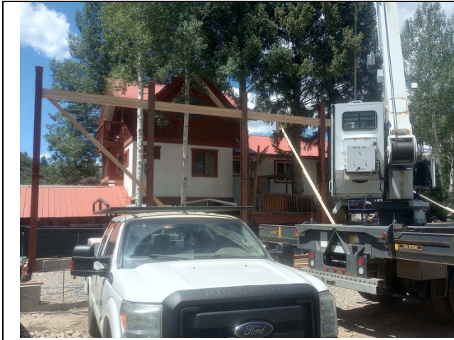
New construction at 491 Main Street.
