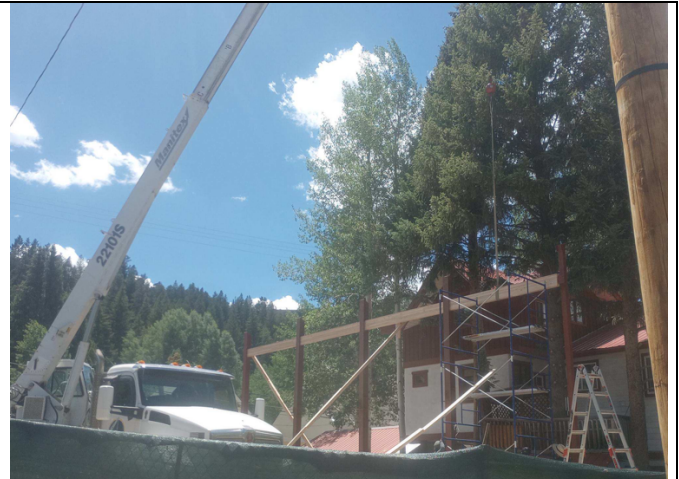
New construction at 491 Main Street.
