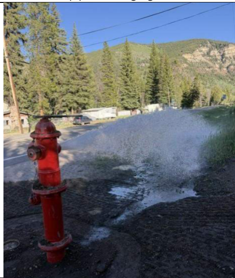
Replaced fire hydrant being flushed.
