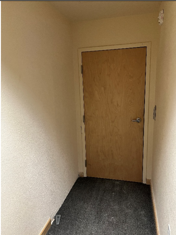
Apartment front door relocated behind secure area.
