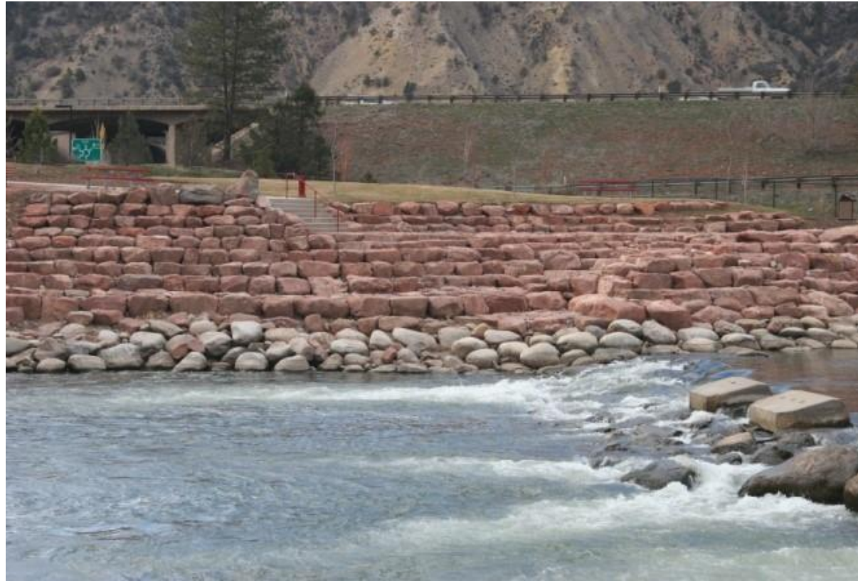
Glenwood Springs Whitewater Park Colorado River, Glenwood Springs, CO 2012 & 2013
