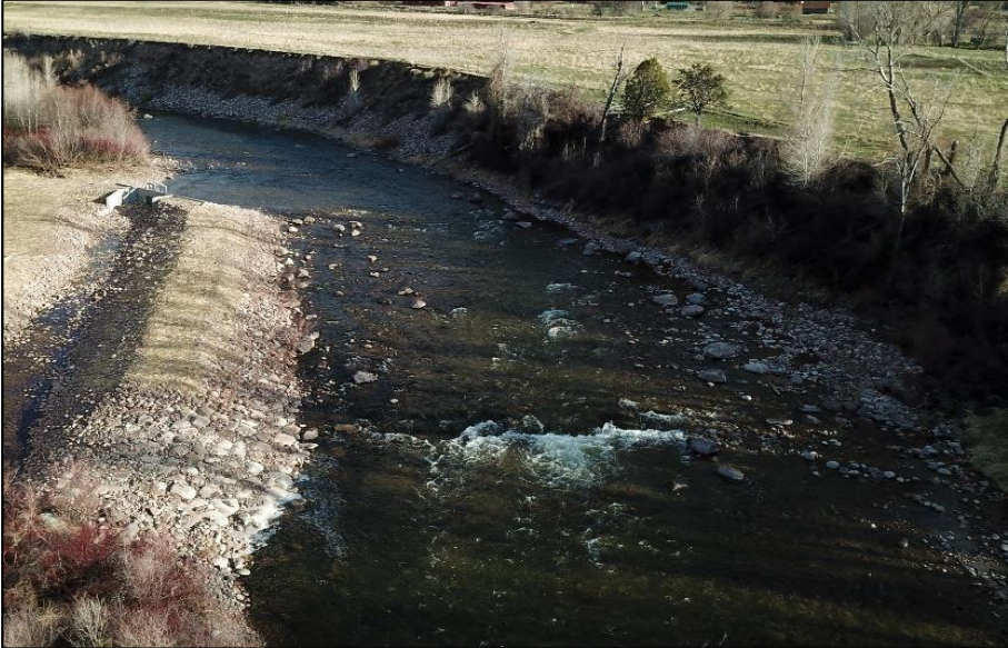
Robinson Diversion post-construction
