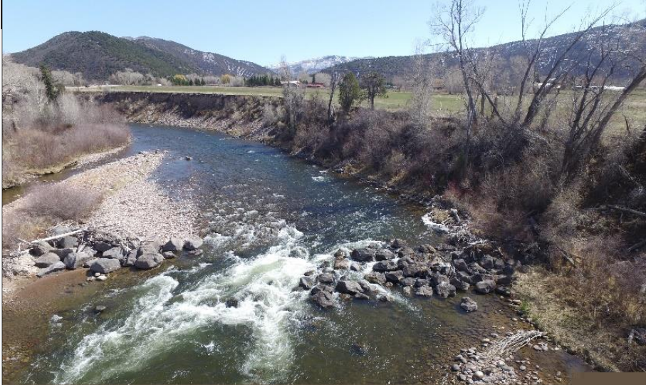
Robinson Diversion structure prior to construction
