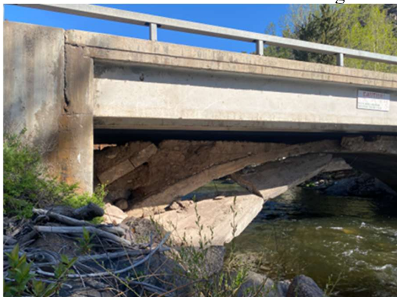
Pictures taken from the south side of the bridge.
