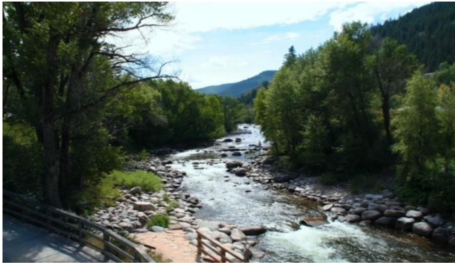
Avon Whitewater Park, Eagle River, Avon, CO 2019 In-channel modification to wave structures
