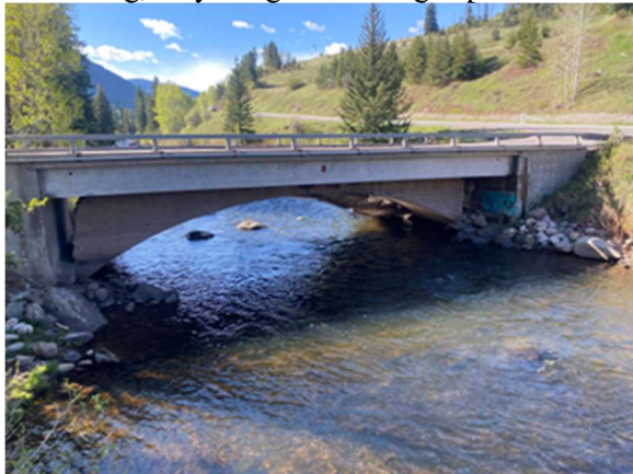
Pictures taken from the north side of bridge.
