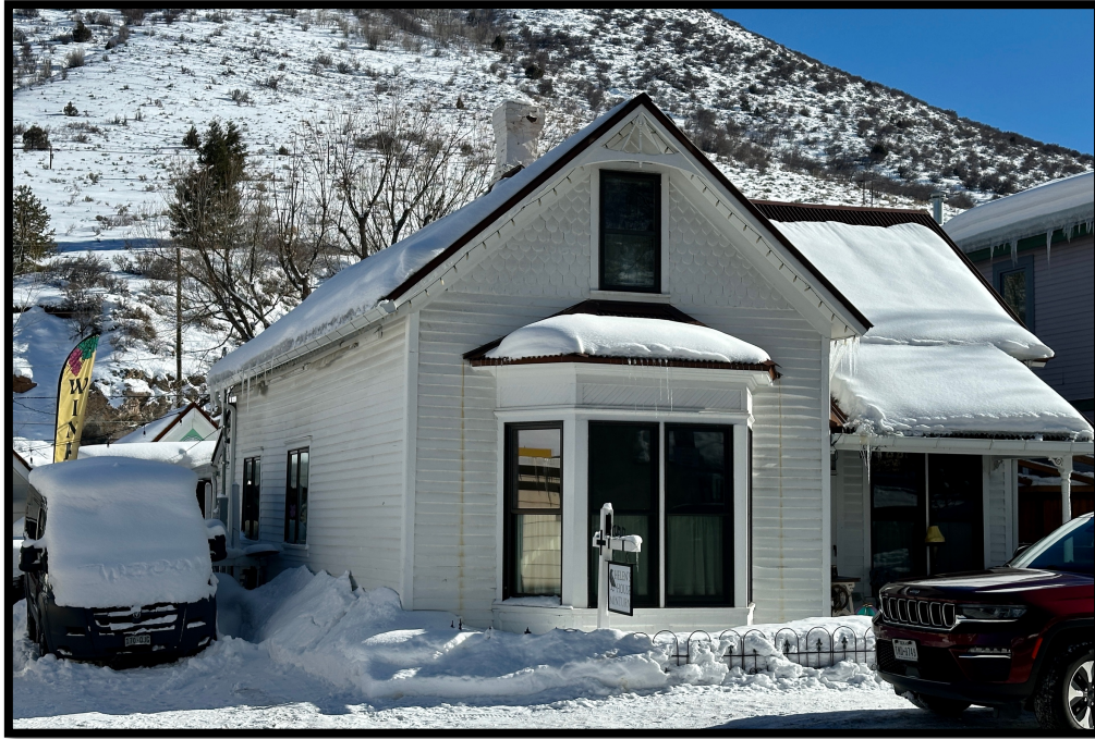
Nelson House, View to the Southeast
