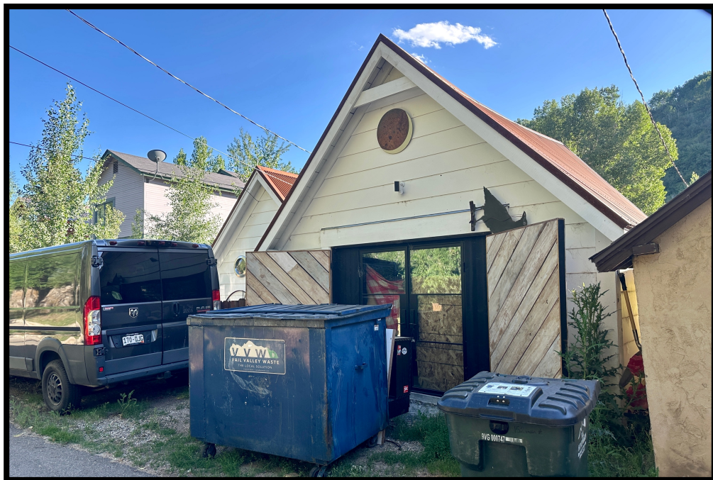
Garage and Milk House, View to the Southwest
