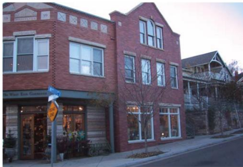
Figure 16-3-#: Scale and Character of New Structures
