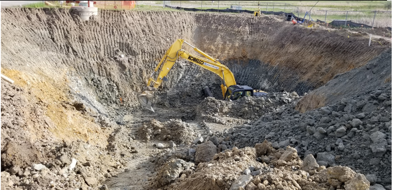
Excavation of the wet and dry wells.
