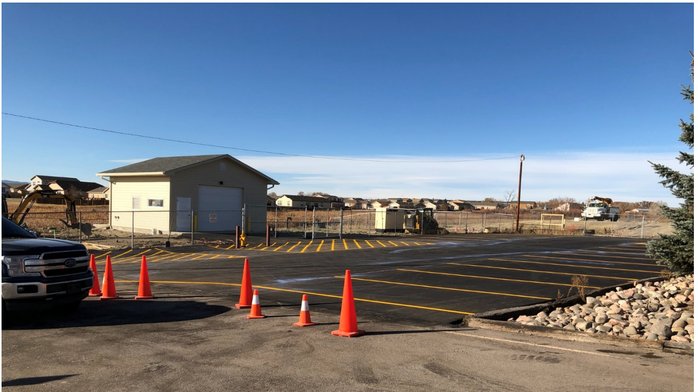
Finalizing the project.
