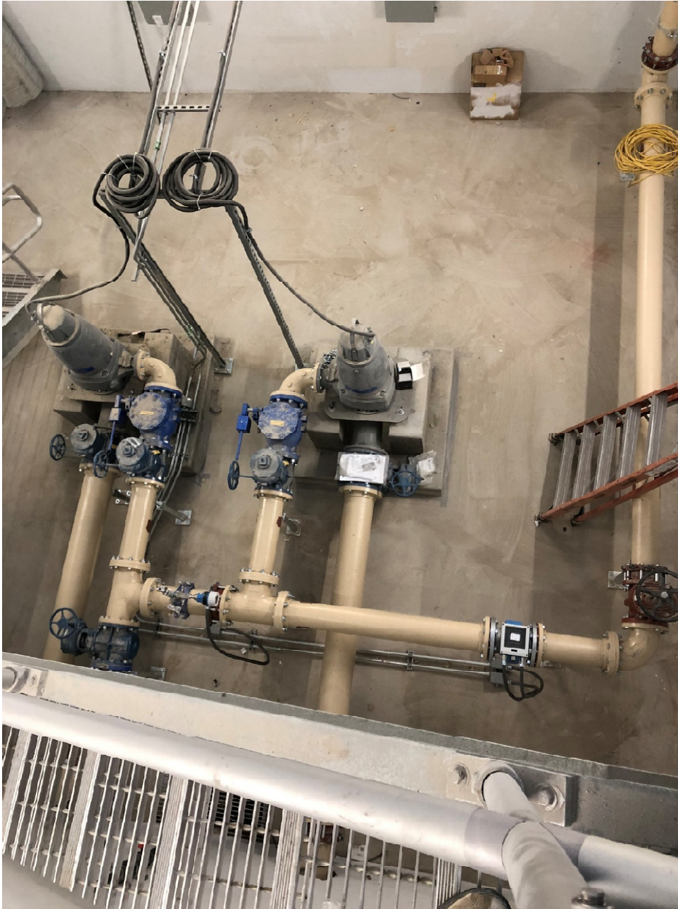
Drywell after pumps were installed.
