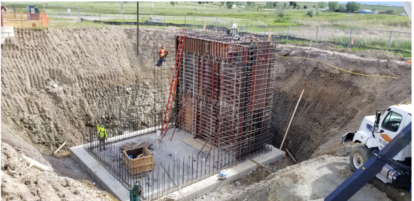
Construction of the wet and dry wells.
