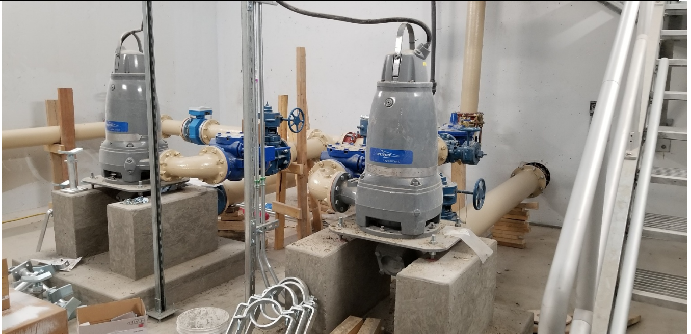
During installation of pumps and process piping.
