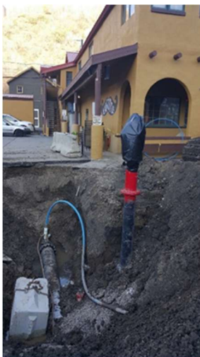
Water Main extension into 1 st Street
