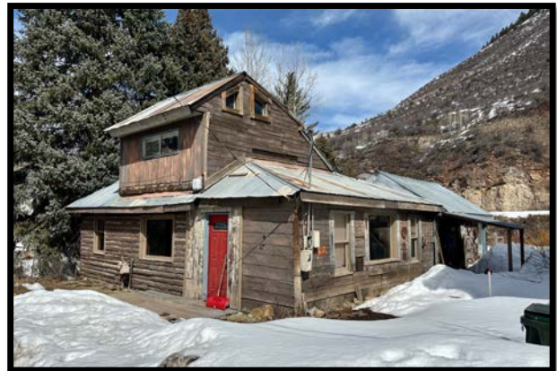
478 Eagle River St., Built 1942 Pioneer Log with Later Additions
