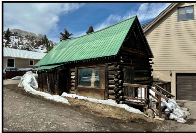
Meyer's Barn, 25 Harrison Ave.
