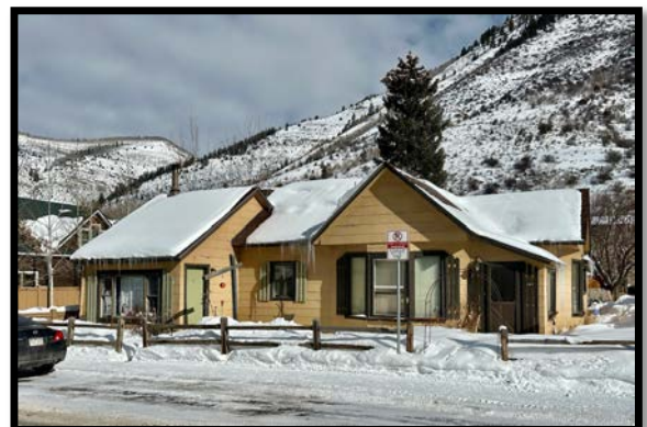
Additions, Non-Original Siding
