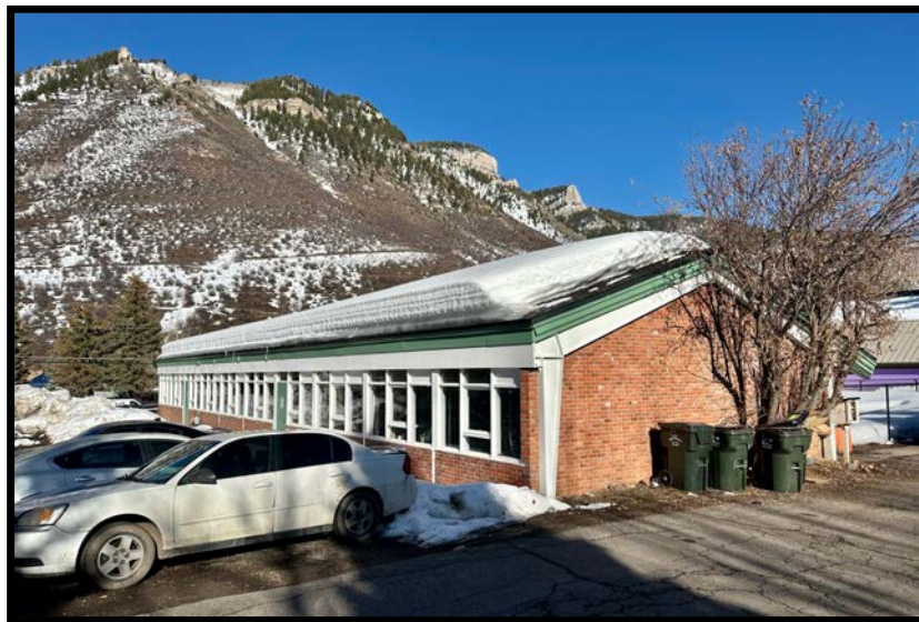
Minturn Elementary School Annex, 423 Pine St. Likely Built in 1956
