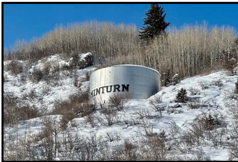
Minturn Water Tank
