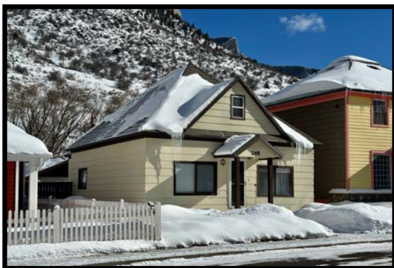
Non-Original Siding, Altered Windows
