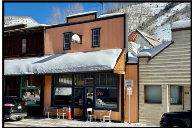
Alterations to Façade, Including Lowered Height of False Front, Siding, Fixed Awning, Upper Windows
