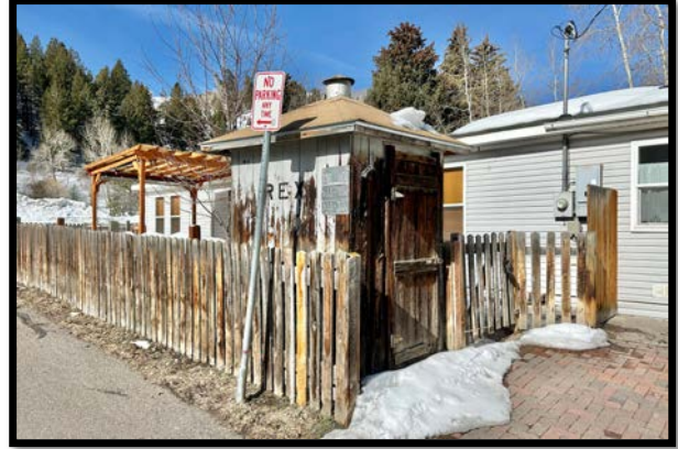
D&RG Railroad, Rex Siding Shed Moved to 470 Pine St.
