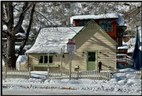
Enclosed Front Porch, Non-Original Siding, Non-Historic Windows
