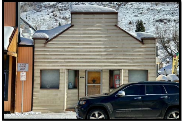
Alterations to False Front, Siding, Storefront Entry and Windows
