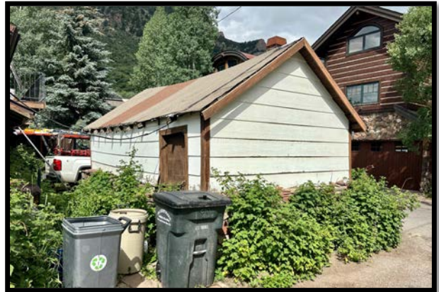
Shed, 591 Main St.
