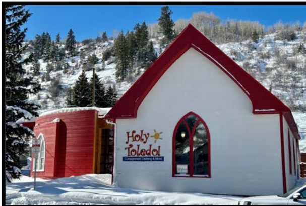
Large Addition, Non-Historic Siding
