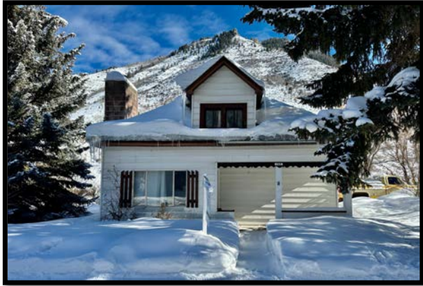
Non-Original Siding, Non-Historic Windows, Non-Historic Chimney
