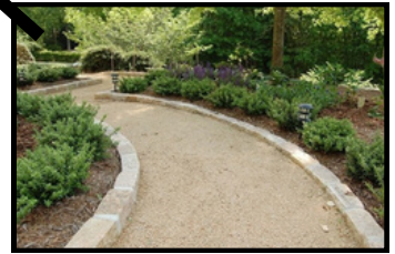
ADA Compliant Stabilized Decomposed Granite Pathway
