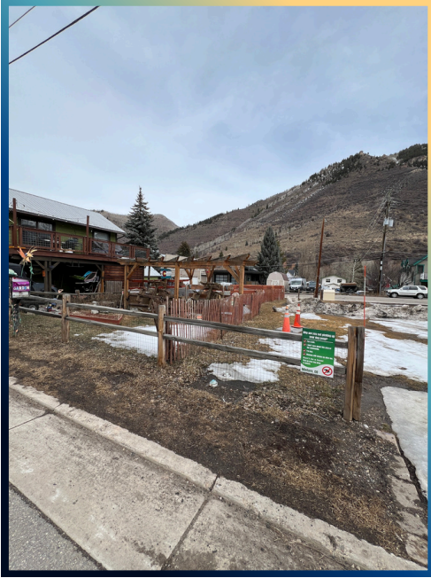
Site Conditions During Winter
