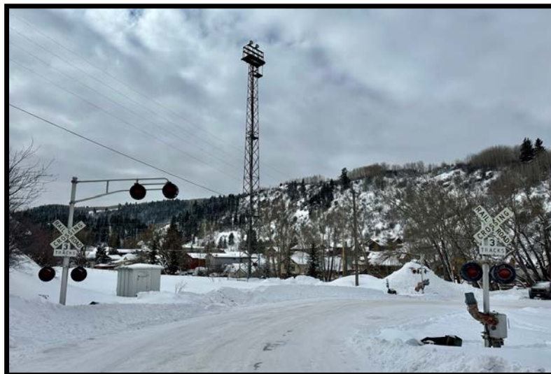
D&RG Railroad Trackside Crossing and Signal Equipment
