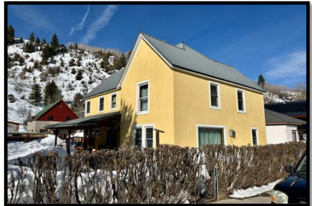
293 Boulder St., Built 1910
