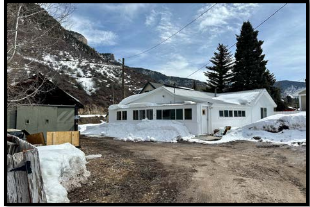
382 Eagle River St., Built 1943
