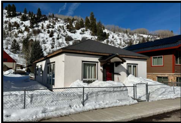
283 Boulder St., Built 1934
