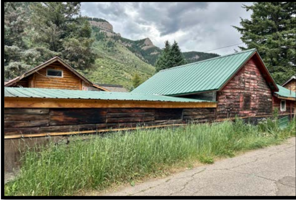
Sheds, 671 Main St.
