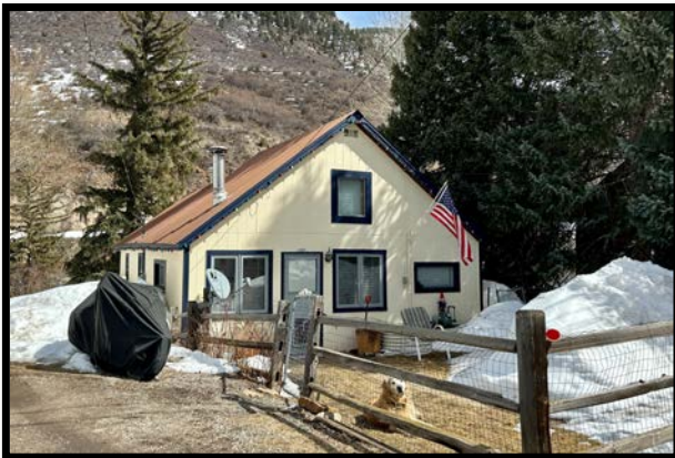
464 Eagle River St., Built 1940
