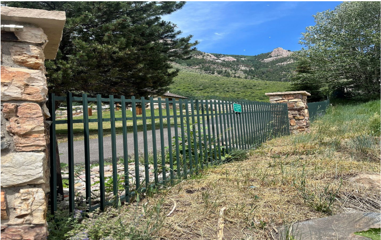
South Side of Fence Section with no Spikes
