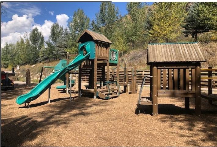
Non-Code Compliant Playground Structure
