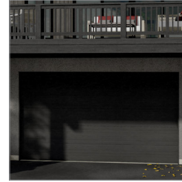
Garage Door 9'-0" x 18'-0" Insulated Metal Color: Black
